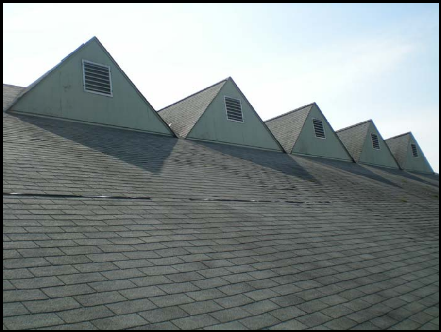
Photo- 1 Overview of the North Roof
