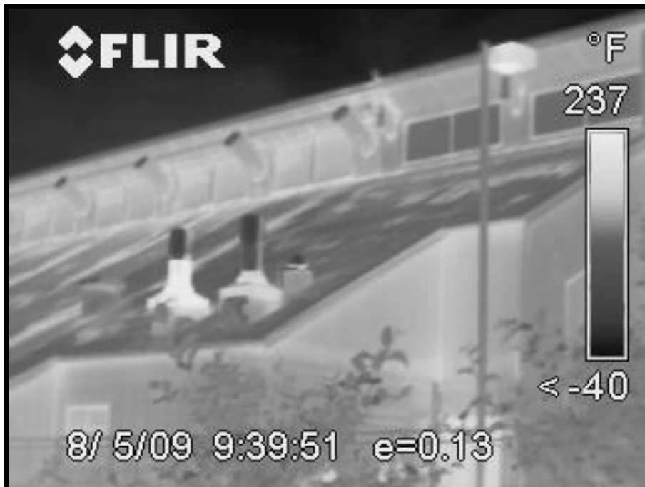
Figure 5 South Elevation Roof Above the Boiler Room
