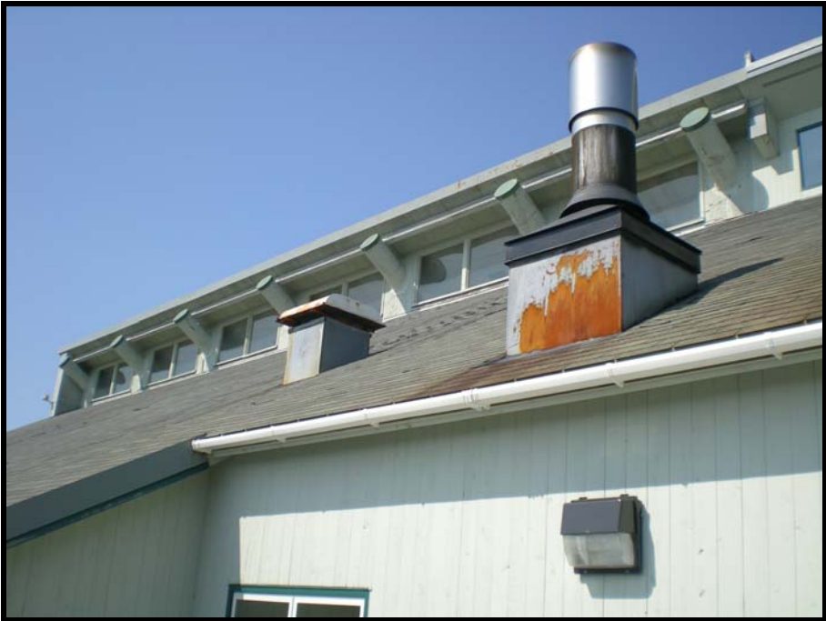
Photo- 2 Overview of the South Roof
