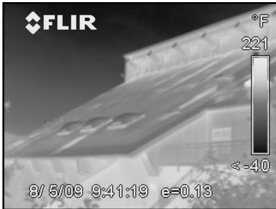
Figure 6 Infrared Photo of Southwest Area of Roof
