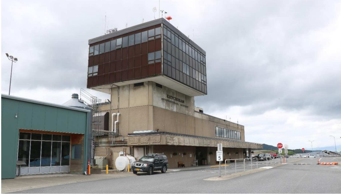
Caption: View of the side (south) elevation and primary facade (landside) of the KTN terminal building and the biomass boiler building from the landside, view facing northwest.
