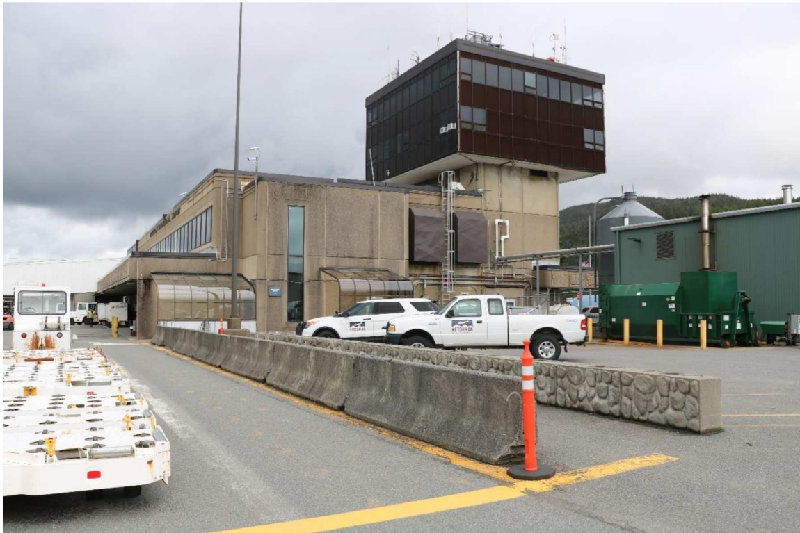
Caption: View of the side (south) elevation and the rear (airside) elevation of the 2016 biomass boiler building from the airside, view facing north.
