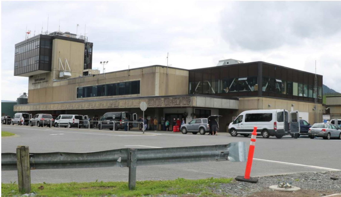
Caption: Overview of the KTN terminal building from the landside, view facing south.
