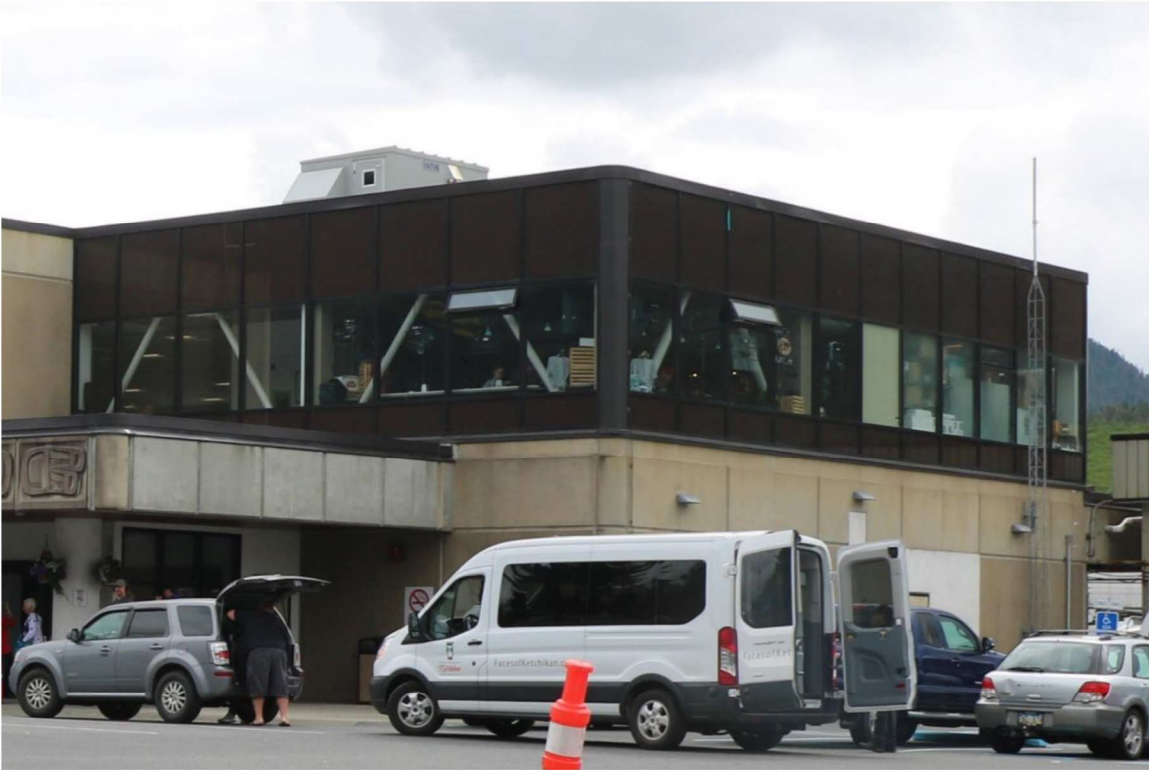
Figure 25. The second-story addition on the north facade of the terminal building, view facing southwest. Mead & Hunt, Inc. July 11, 2022.
