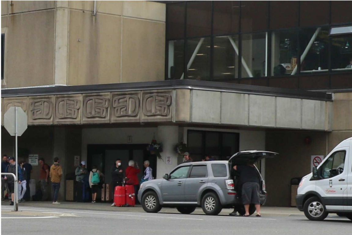
Figure 26. The extended cantilevered awning located at the northeast corner of the terminal building (landside), view facing south. Mead & Hunt photograph, July 11, 2022.
