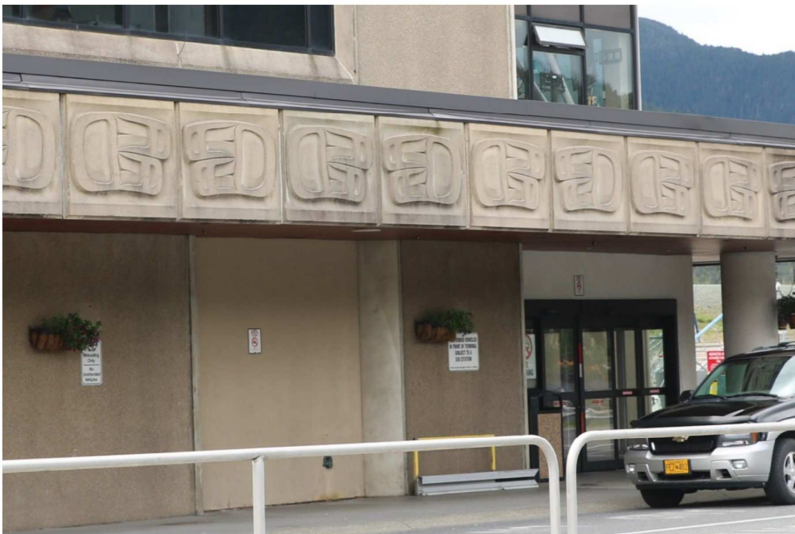
Figure 28. The former northeast corner entrance (now enclosed, red arrow) and the new northeast entrance (blue arrow), view facing northwest. Mead & Hunt photograph July 11, 2022.
