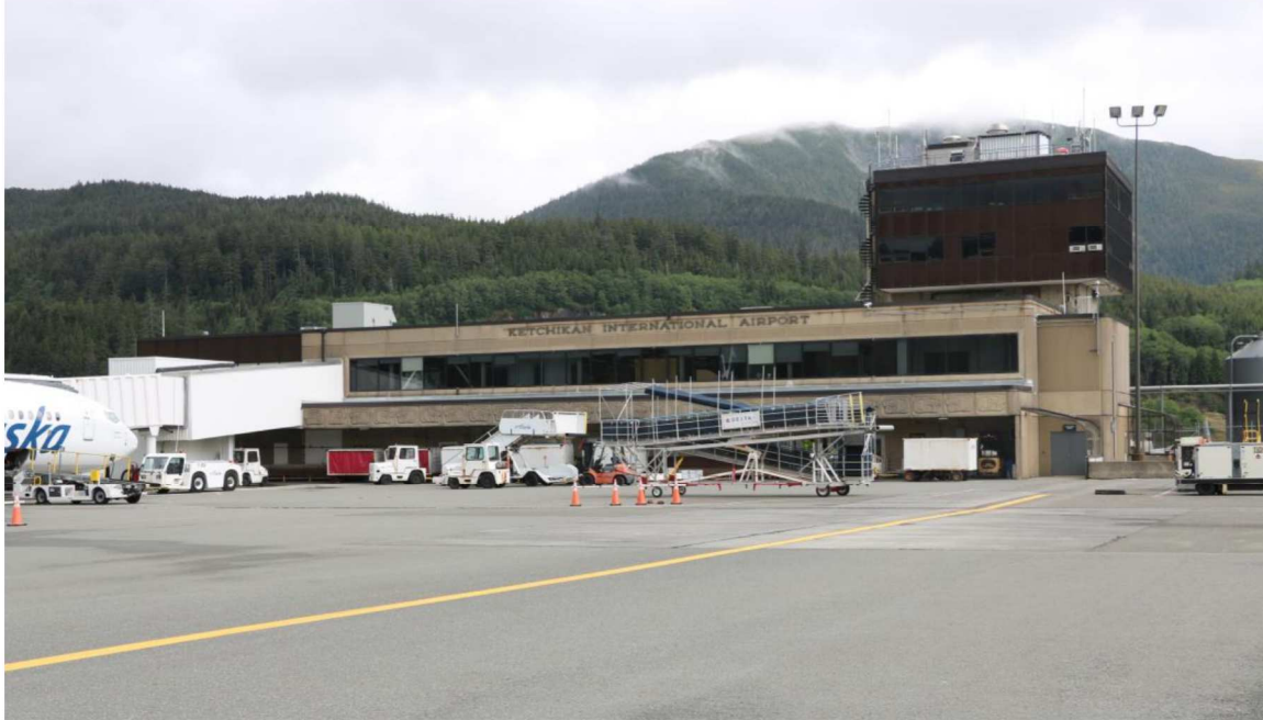
Caption: Overview of the KTN terminal building and apron from the airside, view facing northeast.
