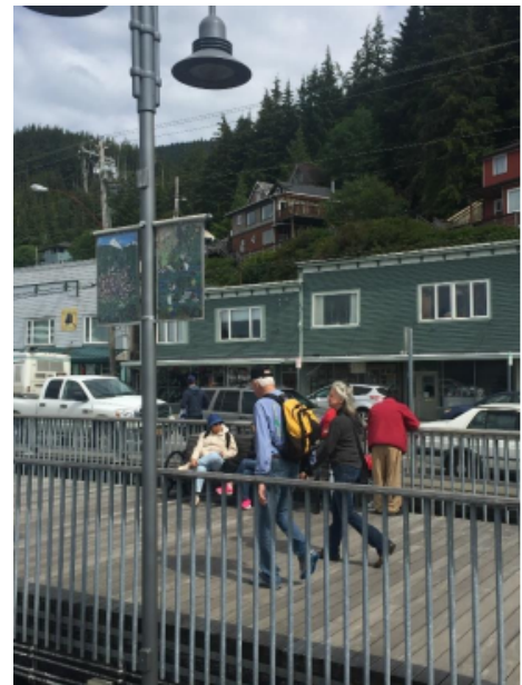
While very visible, the storefronts along Water Street lack sufficient color and historic expression to attract visitors from the SeaWalk.
