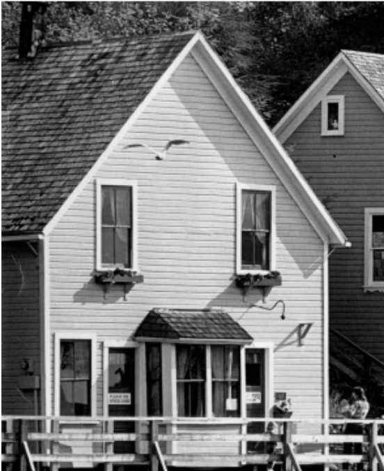
Shortly after restoration in 1976, Dolly's House sports restored siding and window trim and a new cedar shake roof.
