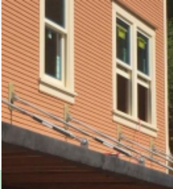
The current restoration of the historic Bayside Hotel (1927) is using a Marvin clad energy efficient window to replicate the original double-hung windows and trim. All original exterior detailing was replicated.
