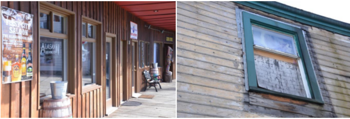
The Water Street facade is a historically appropriate siding (though not original) and the Young Street facade (upper right) still has much of its original siding intact.
