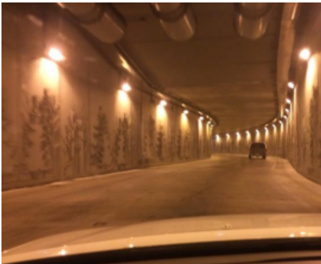
THE VEHICLE TUNNEL AT THE BREMERTON, WASHINGTON FERRY TERMINAL EMPLOYS WALL SCONCES FOR A BRIGHT, INVITING INTERIOR AND THE TUNNEL WALLS ARE "FORESTED" WITH BAS RELIEF OF NORTHWEST TREES TO GIVE A THREE-DIMENSIONAL EFFECT.
