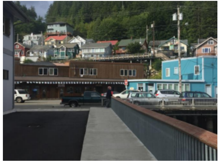
NEW SIDEWALK OPPOSITE THE BAUER WAY ENTRANCE TO HOPKINS ALLEY
