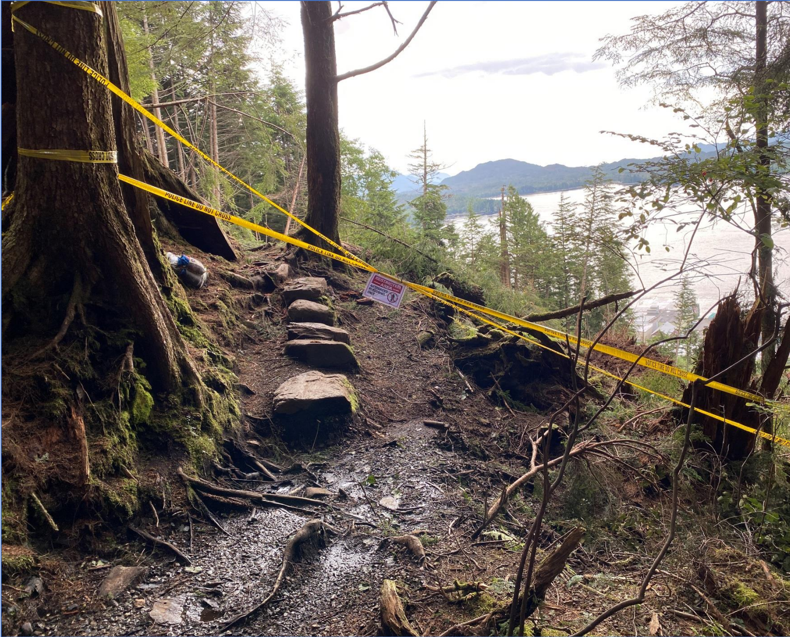
Tape and signs were placed near the slide zone to further discourage individuals from accessing the site. Photo courtesy of AkDoT&PF.
