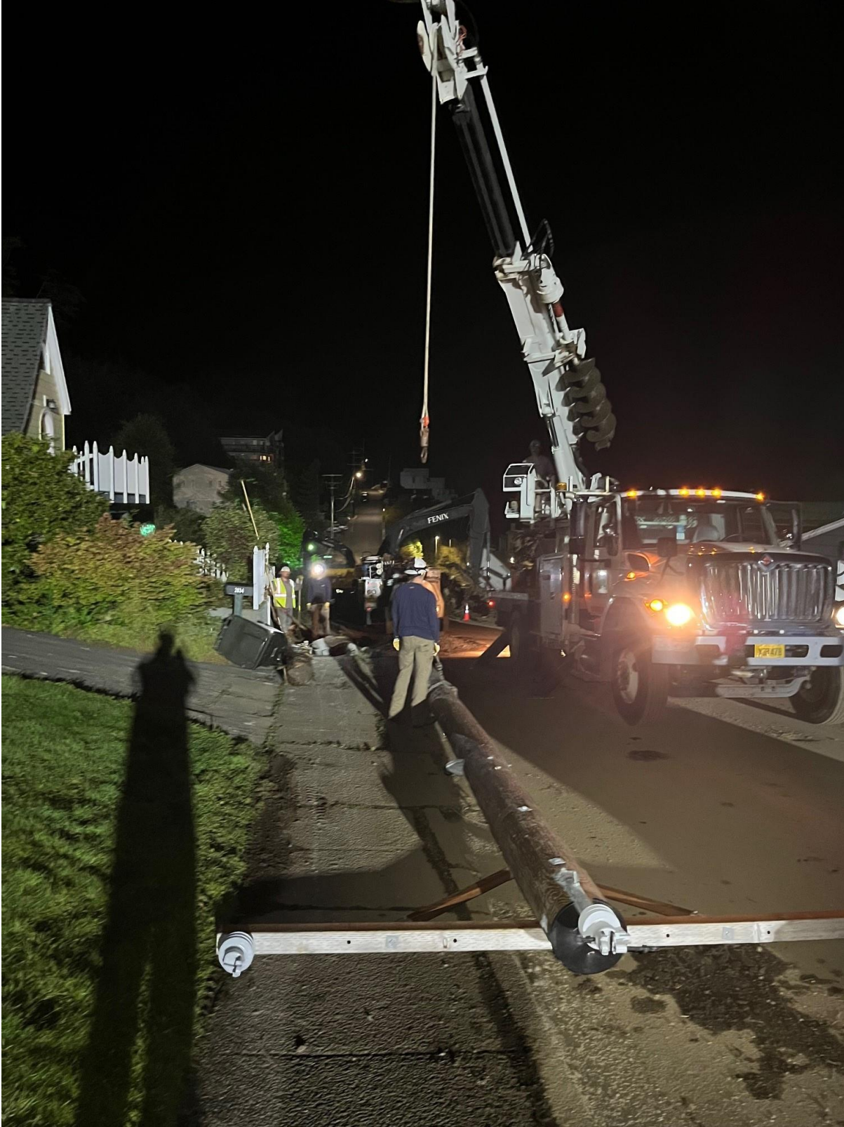
KPU Electric crew installing new electric pole. Photo courtesy of KPU.
