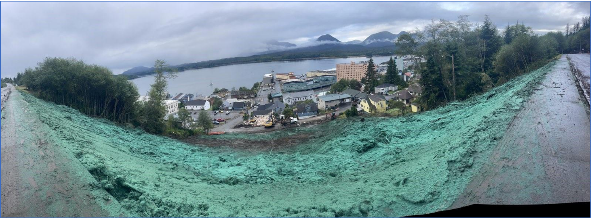
A panoramic view of the freshly hydroseeded slope below the Third Avenue Bypass with the house demolition underway on Whitecliff and Second Avenues below. Photo courtesy of City of Ketchikan.
